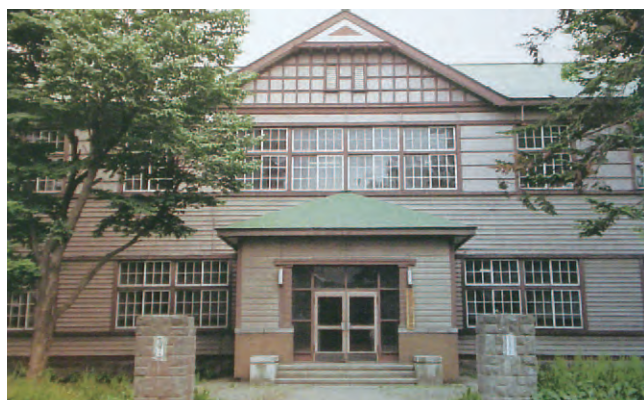
School Building in 1973
